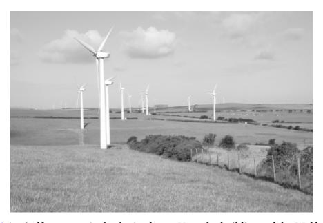
Fig. 15.4 A windfarm near Amlwch, Anglesey. Note the buildings of the Wylfa nuclear power station in the background, on the skyline. The Wylfa power station is in the process of being decommissioned. Wind turbines in the more windy parts of western Britain are erected on shorter masts than their eastern counterparts, where wind speeds are lower.
