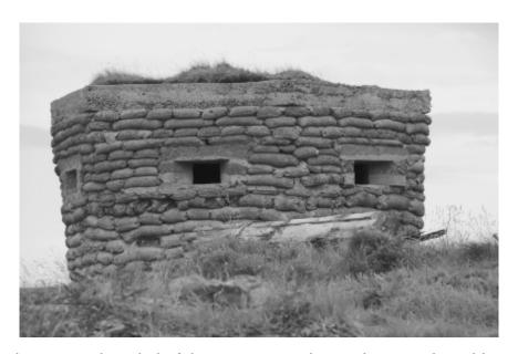
Fig. 14.2 The universal symbol of the Home Front during the Second World War was the polygonal pillbox. This eight-sided example was built near Kirkwall on Mainland Orkney and is most unusual in being made from concrete-filled sacks. This rough exterior would not have deflected incoming shells or bullets very effectively. Note the earth heaped on the roof to provide camouflage against aerial reconnaissance.
