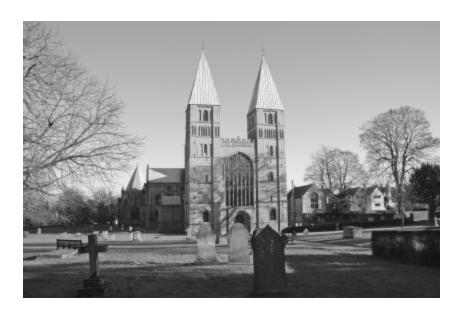
Fig. 8.7 The west front of Southwell Minster, Nottinghamshire. This is one of the finest surviving early Norman minsters in Britain. With the exception of the large Decorated (fifteenth-century) west window, the towers, nave and transept are all Norman work, begun in 1108 and completed fifty years later.
