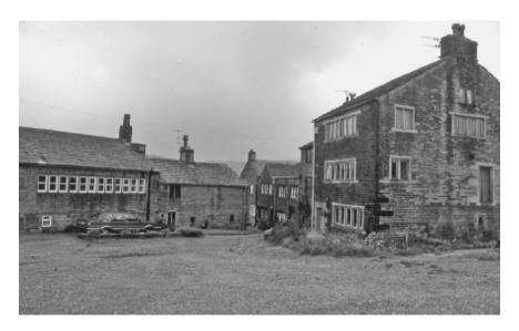
Fig. 13.10 A group of buildings at New Tame Fold, near Saddleworth in Greater Manchester. These workshops are grouped around a farmhouse belonging to a yeoman clothier who supervised the conversion of cloth to clothing. Note the long windows to admit the maximum daylight and the first-floor taking-in door in the gable-end wall of the building to the right; this was where cloth and yarn were brought into the workshops, from handweavers in the region.
