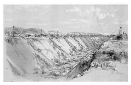
Fig. 13.3 Navvies digging the Tring (Hertfordshire) cutting on the London and Birmingham railway, June 1837. Note the steep, planked barrow runs. Sometimes barrows would be
