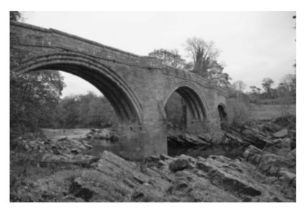
Fig. 9.17 The Devil's Bridge, Kirkby Lonsdale, Cumbria. The three arches of this fifteenth century bridge carry the road to Ingleton across the River Lune. Many upland medieval bridges have been swept away when rivers were in spate, but this fine example has survived because its piers were placed high, on solid outcrops of rock.
