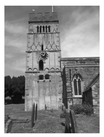
Fig. 7.10 The Saxon tower of All Saints church, Earls Barton, near Wellingborough, Northamptonshire. The tower is superbly decorated in the later Saxon style, with so-called 'long-and-short work' at the corner angles and raised bands of stone often said to imitate woodwork.
