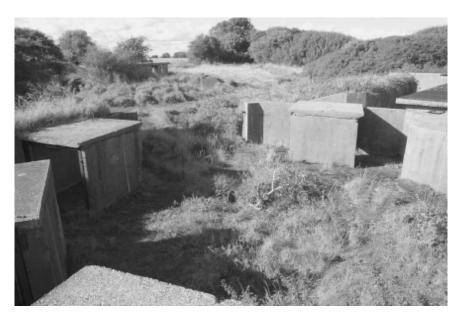
Fig. 14.5 Heavy anti-aircraft battery at St Margaret's-at-Cliffe, near Dover, Kent. The anti-aircraft gun would have been mounted at the centre of this circular arrangement of slab-built concrete ammunition lockers. In the background is the battery command and communication centre. Heavy anti-aircraft batteries were established along the south coast to protect London from bombers and later from V1 flying bombs launched in Holland and France.
