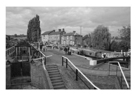
Fig. 11.14 The Grand Union Canal at Stoke Bruerne, Northamptonshire, showing the parallel locks. The original (1805) lock is to the left (today it is blocked off and used as a dry dock). The new parallel lock is to the right and is still in active use; it was added in 1835–40 to speed traffic in an ultimately unsuccessful attempt to compete with the emerging railways.
