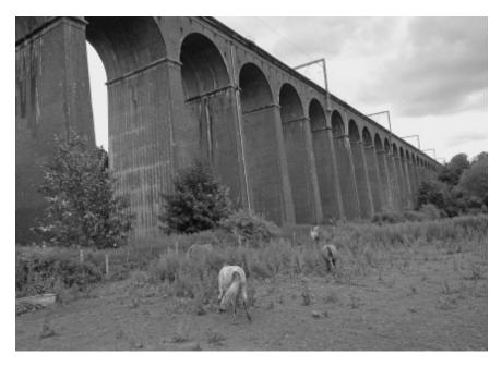
Fig. 13.1 The Digswell Viaduct, near Welwyn, Hertfordshire. This viaduct carries two tracks of the Great Northern railway over the steep-sided valley of the River Mimran. It has fortynine brick arches, each with a span of 9.1 metres, and was built between 1848 and 1850. The engineer was Lewis Cubitt (1811–72), and the construction was the work of Thomas Brassey (1805–70), who built about a third of Britain's early railways with great efficiency – usually to budget and to time.
