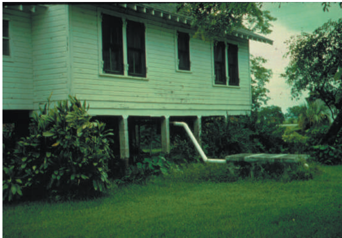
Figure 3.24 Soil subsidence due to rapid organic matter decomposition after artificial drainage of Histosols in the Florida Everglades, USA. The house was built at ground level, with the septic tank buried about 1 m below the soil surface. Over a period of about 60 years, more than 1.2 m of the organic soil has “disappeared.” The loss has been especially rapid because of Florida’s warm climate, but artificial drainage that lowers the water table and continually dries out the upper horizons is an unsustainable practice on any Histosol. (Photo courtesy of George H. Snyder, Everglades Research and Education Center, Belle Glade, FL)
