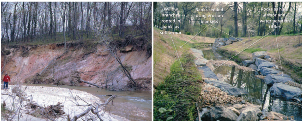
Figure 17.39 Stream bank erosion and its control with bioengineering techniques. (Left) Tumbling trees are a sign of a degraded stream with rapidly eroding banks that contribute large amounts of soils to the stream sediment load. (Right) A somewhat smaller stream that was similarly degraded, but has now been restored with several techniques that control bank erosion and improve water quality. The banks have been protected from scouring storm flows by both soft armor and hard armor. As soft armor, the stream banks have been seeded with a diversity of native grasses and forbs and the seeding protected temporarily by biodegradable erosion blankets. The live willow branches that are taking root along the base of the stream banks comprise another type of soft armor referred to as live staking. The large rocks (hard armor) protect the banks from scouring, cause water to form rapids that improve water oxygen content, and collect gravelly sediments that improve fish-spawning habitat. (Photos courtesy of Ray R. Weil)
