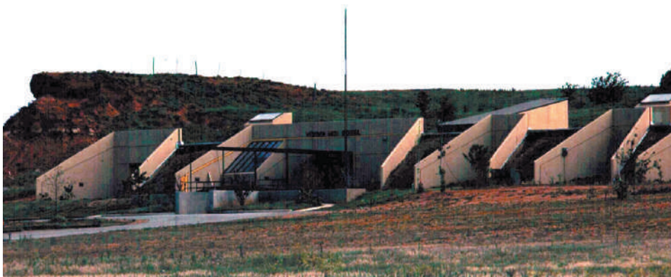
Figure 7.37 This high school in Oklahoma, USA, has been built into the ground with only one side exposed. This design takes advantage of the high specific heat and low thermal conductivity of the overlying soils, keeping the school warm in winter and cool in summer with a minimum of energy used for heating or air-conditioning.
