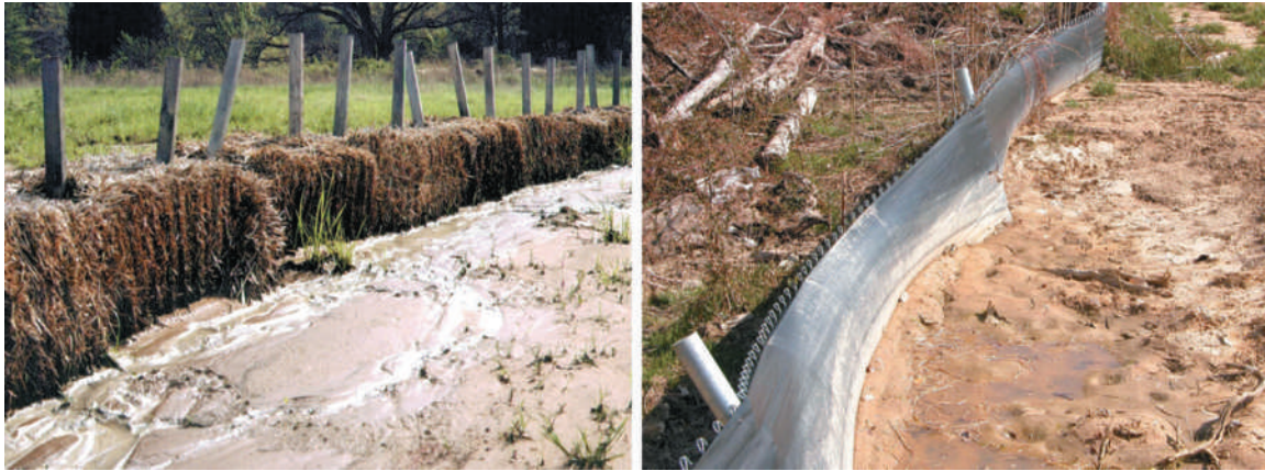
Figure 17.40 Several types of sediment-control measures used around the periphery of a construction site. (Left) A line of straw bales pegged to the ground allows water to seep through, but filters out much of the sediment and slows down the flow so that the water drops its sediment load. (Right) A properly installed silt fence effectively removes sediment from runoff water leaving the edge of a construction site. The silt fencing material is a woven plastic that allows water to flow through at a much reduced rate. Note the light-colored sediment on the inside and the undisturbed forest floor on the outside of the silt fence. A silt fence must be embedded in the soil and supported with stout stakes or posts. Improperly installed silt fencing is useless, as sediment-laden water may pass underneath or may even knock the fence over. (Photos courtesy of Ray R. Weil)
