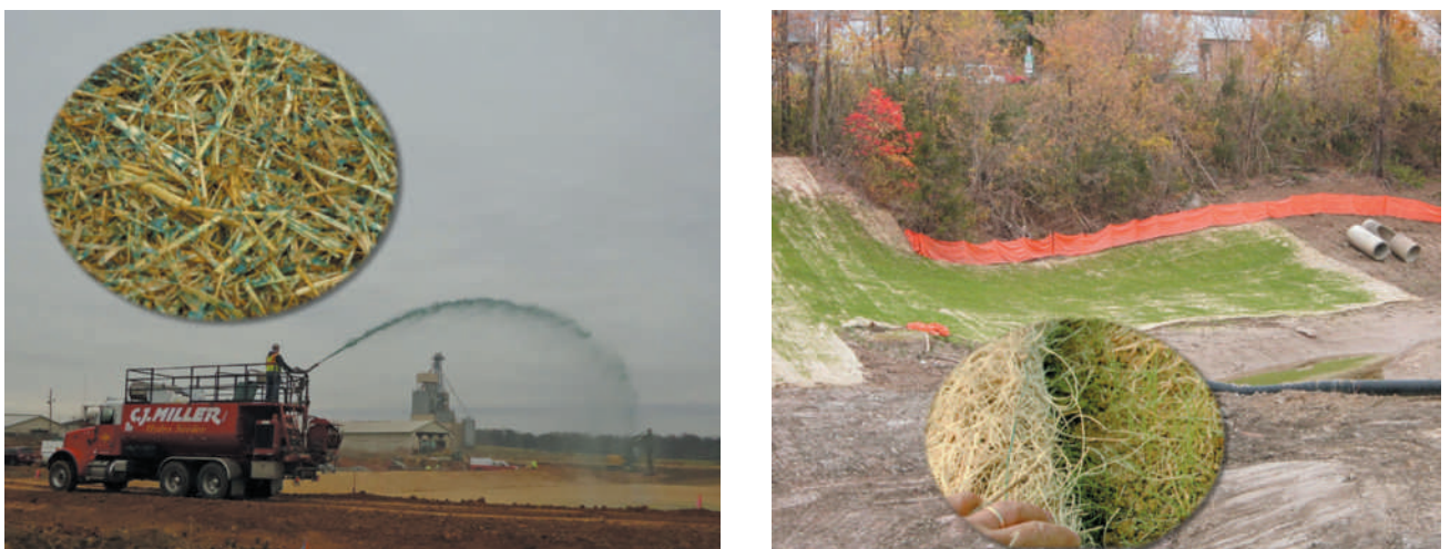
Figure 17.36 Two means of providing rapid temporary soil cover while establishing vegetation on erodible slopes. (Left) A hydroseeder spraying a mixture of water, chopped straw, grass seed, fertilizer, and sticky polymers (inset close-up) that holds the mulch in place until the grass seed can take root. Hydroseeding is especially useful for efficiently establishing vegetative cover on difficult-to-reach areas. (Right) Erosion-control mats or blankets made of plastic netting or natural materials like wood fiber or jute (shown here) are rolled out over newly seeded grass to hold the seed and soil in place until the vegetative cover is established. In the inset, young grass seedlings are exposed as the jute erosion blanket is pulled away. (Photos courtesy of Ray R. Weil)
