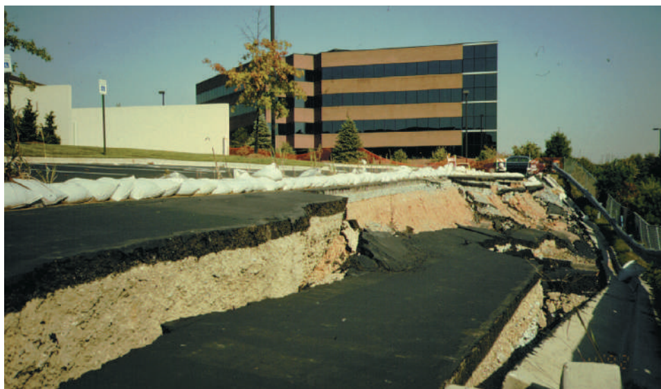
Figure 1.11 Better knowledge of the soils on which this road was built may have allowed its engineers to develop a more stable design, thus avoiding this costly and dangerous situation. (Photo courtesy of Ray R. Weil)
