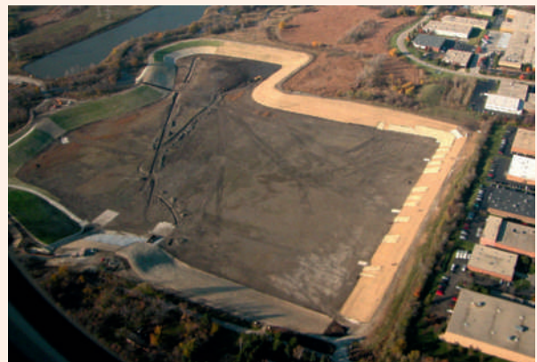
Figure 8.14 A large waste lagoon under construction is being lined with a layer of dark-colored smectitic clay. The very low hydraulic conductivity of the expansive clay will seal in the stored liquid and retard percolation of polluted water. The high CEC of the clay will retard leaching of pollutants by retaining dissolved pollutants, even when some water movement takes place. Straw-colored erosion blankets are also being used to establish erosion controlling grasses on the berms. (Photo by Ray R. Weil)
