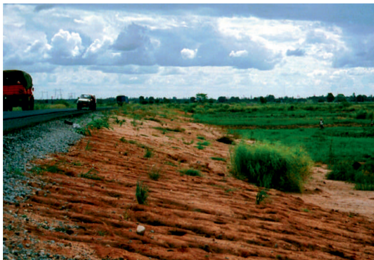
Figure 8.7 A road in southeastern Tanzania crossing a large valley comprised of black soils high in expansive 2:1 clays. A stable roadbed was built up by trucking the red colored soil material seen in the foreground. This soil material came from distance uplands where the soils were better drained, more weathered, and dominated by the 1:1 clay mineral kaolinite. The black soils adjacent to the road would have been much more conveniently and inexpensively used, but their high content of 2:1 clays made them completely unsuitable for a road base. The 2:1 clays shrink in dry weather and swell up in wet weather and thus would have caused rapid heaving and cracking of the pavement. (Photo courtesy of Ray R. Weil)
