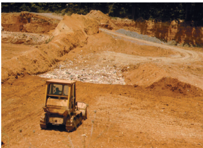
Figure 18.35 A bulldozer compacts and buries trash in an old natural attenuation landfill in deep, well-drained soils. The trash is covered daily by 15 cm of soil to prevent it from being carried away by wind or infested with rats. Once the entire trench is filled, a much thicker final cover of soil will be applied. Note the lack of any geomembrane liner or leachate collection system in this landfill. (Photo by Ray R. Weil)
