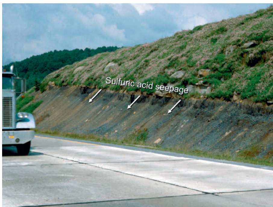
Figure 13.53 Construction of this highway cut through several layers of sedimentary rock. One of these layers contained reduced sulfide materials. Now exposed to the air and water, this layer is producing copious quantities of sulfuric acid as the sulfide materials are oxidized. Note the failure of vegetation to grow below the zone from which the acid is draining. (Photo courtesy of Ray R. Weil)
