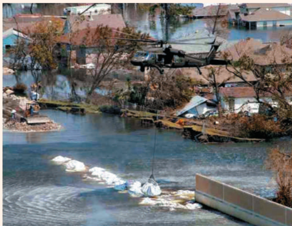
Figure 4.64 A large helicopter attempts emergency repairs to the 17th Street levee breach several days after Hurricane Katrina hit New Orleans and toppled this section of the levee and seawall. Large chunks of the levee can be seen some 14 m inland. (Photo courtesy of U.S. Army Corps of Engineers)
