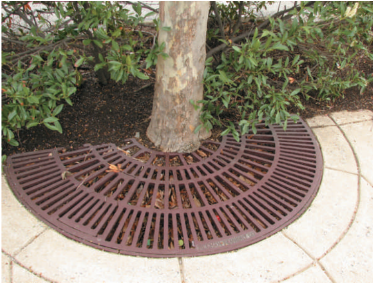
Figure 4.49 A cast iron grill designed to protect a young urban tree root zone from compaction by foot traffic while allowing rain water and air to readily penetrate into the root zone. The concentric circles of grillwork are designed to be broken off to enlarge the trunk hole before girdling can occur. Unfortunately, in this case maintenance has been lax, so the trunk has outgrown the hole and the grill is starting to girdle the tree. (Photo courtesy of Ray R. Weil)
