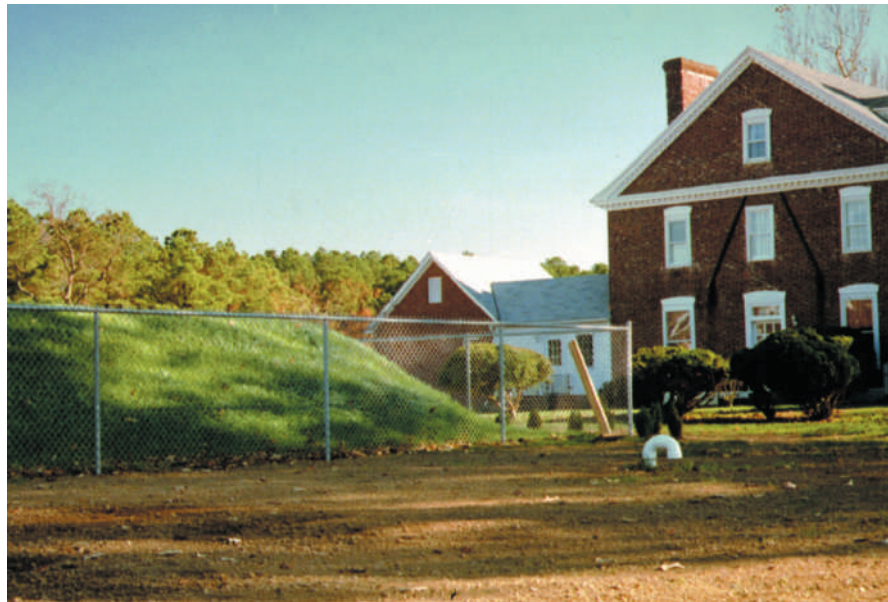
Figure 6.45 A mound-type septic tank effluent treatment system installed for an historic house in a flat, poorly drained region where the shallow water table precludes the burial of septic drain lines in conventional deep ditches. Note the white air vent pipe at the foot of the mound in the foreground. (Photo courtesy of Ray R. Weil)
