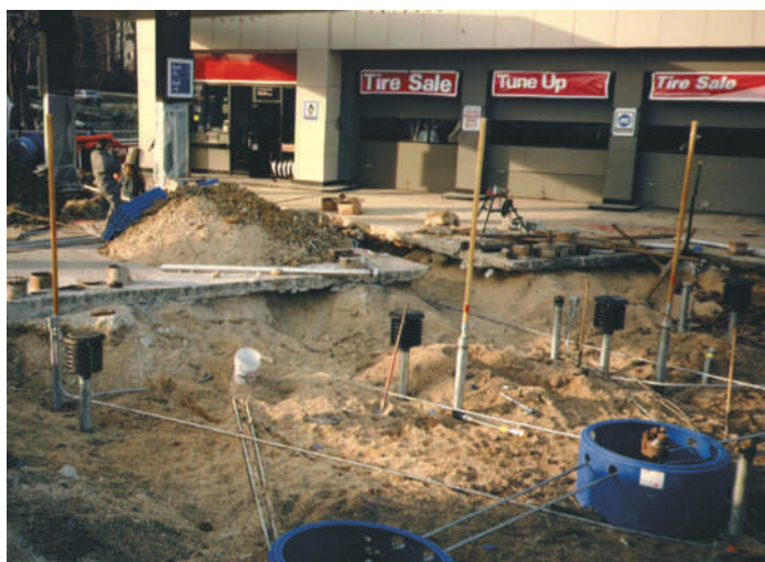
Figure 18.3 Leaking underground storage tank (LUST) replacement at a gas station in California, USA. The old rusting steel tanks have been removed and replaced by more corrosion-resistant fiberglass tanks, which are set in the ground and covered with pea gravel. The soil and groundwater aquifer beneath the tanks were cleaned up using special techniques to stimulate soil microorganisms and to pump out volatile organics such as benzene vapors. Remediation and replacement can cost about $1 million for a single large gas station. (Photo courtesy of Ray R. Weil)
