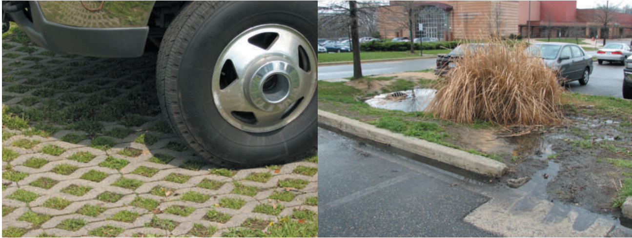
Figure 6.13 Two methods of increasing infiltration and slowing runoff in urbanized watersheds. (Left) Permeable pavers allow grass to grow and water to infiltrate a parking lot while cars can still park without compacting soil or forming mud. (Right) Water entering one of several small rain gardens that capture runoff from a suburban parking lot. The water is directed to a small depression. The small pond that forms is ephemeral, holding the runoff water only temporarily. Permeable soil placed under the depression along with buried drain pipes are designed to allow the water to infiltrate and seep away over a period of a few hours. The depression is planted with a variety of native plants that provide both beauty and wildlife habitat. (Photos courtesy of Ray R. Weil)
