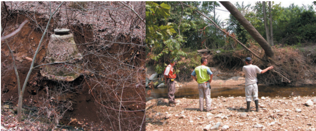
Figure 6.12 Signs of excessive runoff from urbanized land. (Left) Exposure of a once-buried storm sewer manhole along a highly degraded stream that collects runoff from part of Baltimore in Maryland, USA. The drastically increased storm runoff volume from the largely impermeable urban watershed has caused the stream to erode its banks and deeply cut into the hillside. The round manhole cover indicates the former land surface. (Right) The toppled tree and scoured soil are signs that this placid appearing small stream is overwhelmed by raging torrents of water during heavy rainfalls because the urbanized watershed conducts the water more directly and rapidly to the stream than did the natural watershed that formed the stream.
