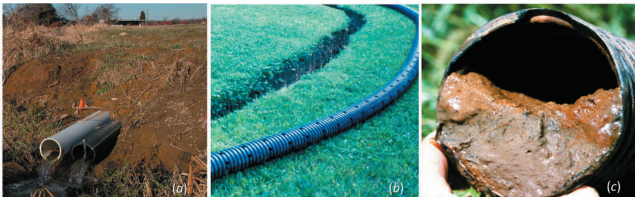
Figure 6.42 Subsurface “tile” drainage systems. (a) Two outlet pipes empty drainage water from a tile drain system into an open ditch. Such an outlet is essential for a gravity drainage system to function. (b) Flexible plastic drainpipe perforated with holes on one side. These holes must be on the bottom of the drainpipe when it is installed, to avoid soil entering and clogging the pipe as shown in (c), where the pipe was installed with the holes on the top. (Photos courtesy of Ray R. Weil)
