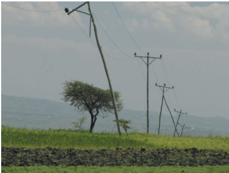
Figure 3.32 Utility poles appear to stagger drunkenly across a Vertisols landscape. The poles are leaning every which way because they are set into Vertisols that contain over 60% clay of a type that swells up when wet but cracks deeply and shrinks as it dries. As a result, the soil shifts or rocks back and forth with the seasons. This shrink–swell action of Vertisols makes them problematic for all kinds of construction. (Photo courtesy of Ray R. Weil)
