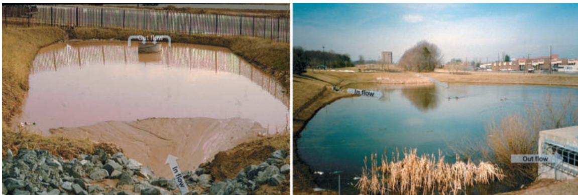
Figure 17.41 Sediment and storm water retention. (Left) The effect of a small sediment impoundment structure on the retention of suspended soil eroded from a construction site. Note the riprap-lined channel leading runoff water into the pond and the delta-like alluvial fan of sediment deposited as the water's velocity is reduced where it enters the pond. The standpipe in the background has holes that allow the clearest water near the top to overflow and leave the construction site. (Right) A larger sediment retention pond shown several years after construction activities were completed. A well-designed sediment structure will serve as a decorative landscaping asset to the property and continue to detain storm water and retain sediment. Only rarely does enough water accumulate to reach the outflow grating, and even then, most sediment is retained on the pond bottom.
